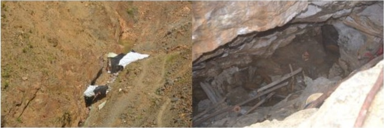
Figure 23: Underground workings Poeketi (October 6, 2022)
